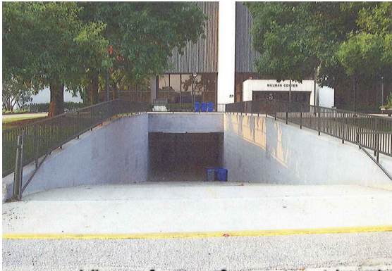
View of ramp from street level
