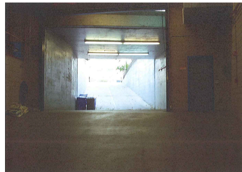
View of ramp from street level
